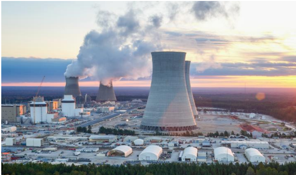
Vogtle Electric Generating Plant Waynesboro, Georgia (USA)
